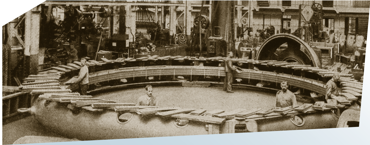
Stacking work on a DC machine in the large machine hall at Sachsenwerk
