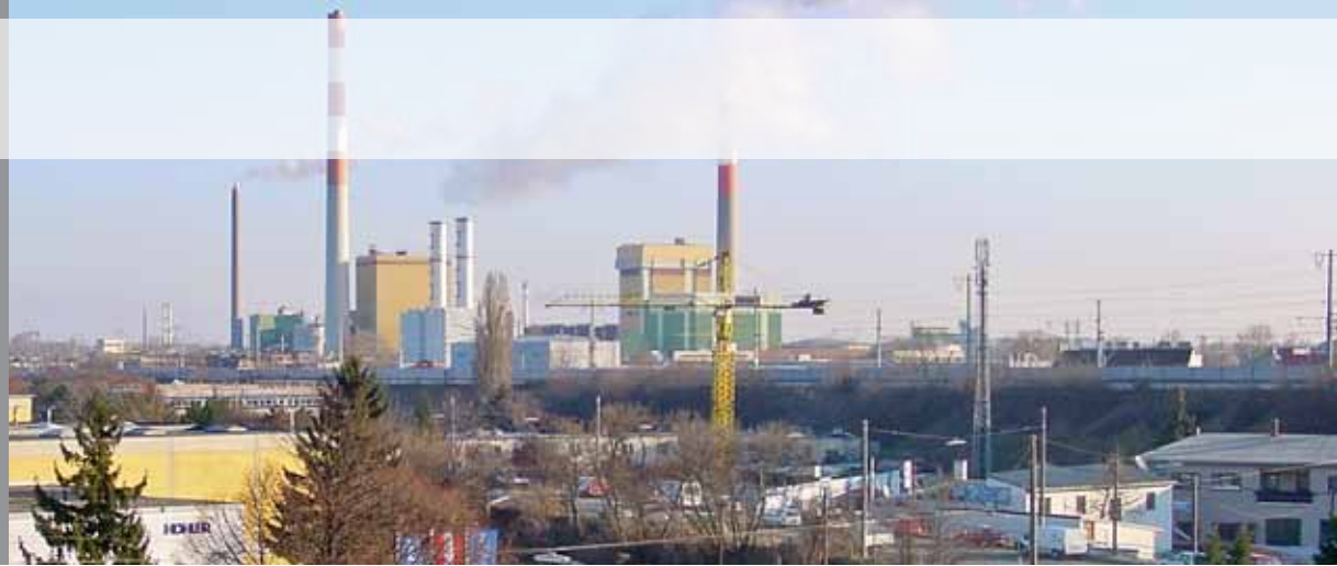
The combined heat and power plant Simmering 3 in Vienna is the largest power plant in Austria.
