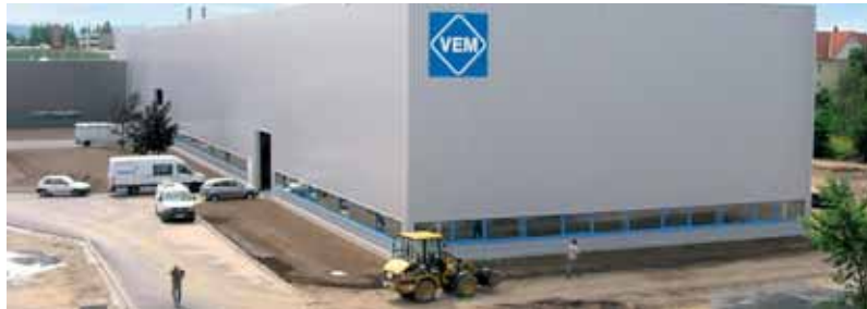
The new hall at Sachsenwerk will be ready for occupation at the end of August 2007.
