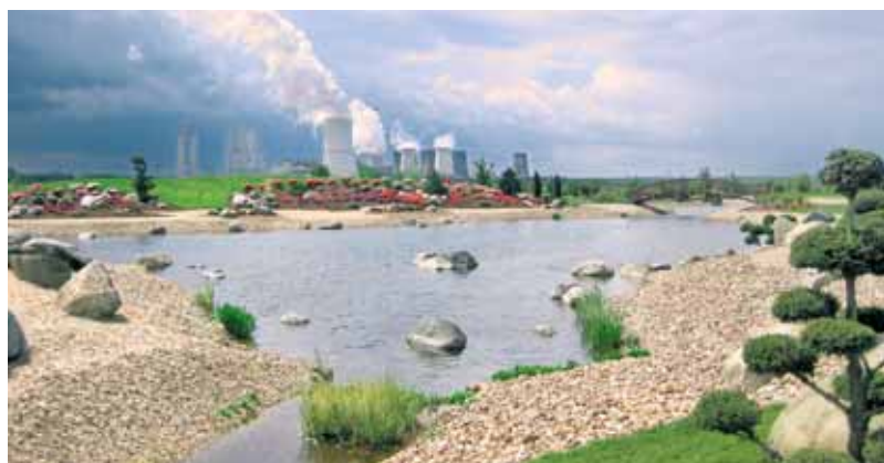
The efficient handling of electrical energy, environmental awareness and careful use of our natural resources were also key topics for the EEMODS conference. Our photo shows the Boxberg power station in Eastern Saxony from the perspective of the newly established Nochten Boulder Park, a former open-cast mining area.
