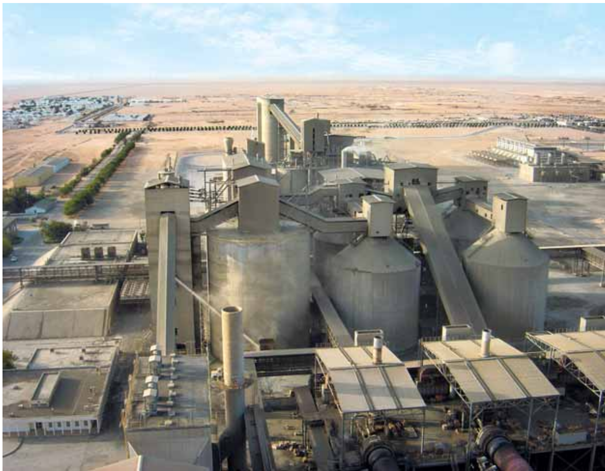
The booming economy in Saudi Arabia is demanding enormous quantities of cement. This new production line has been designed to deliver some 7,000 tonnes of clinker per day.
