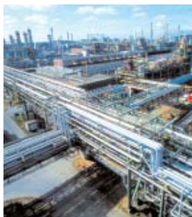
Infrastructure in the Marl Chemical Park
