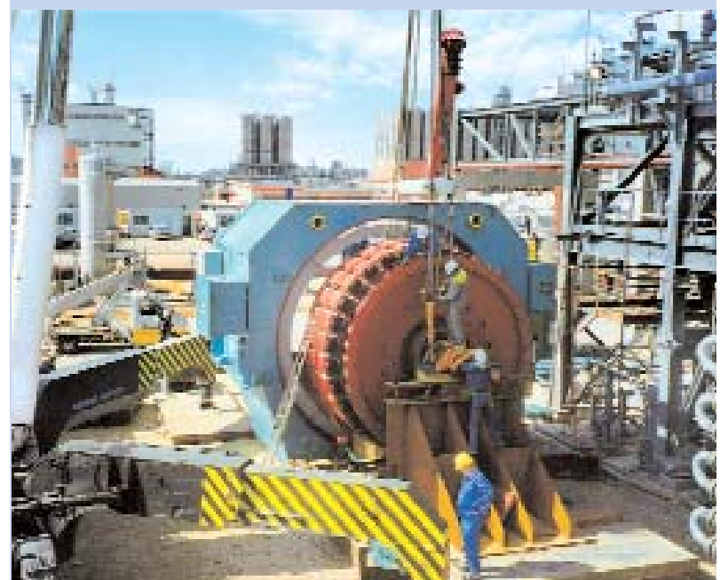
The 160-tonne main compressor drive is lifted into place by crane
