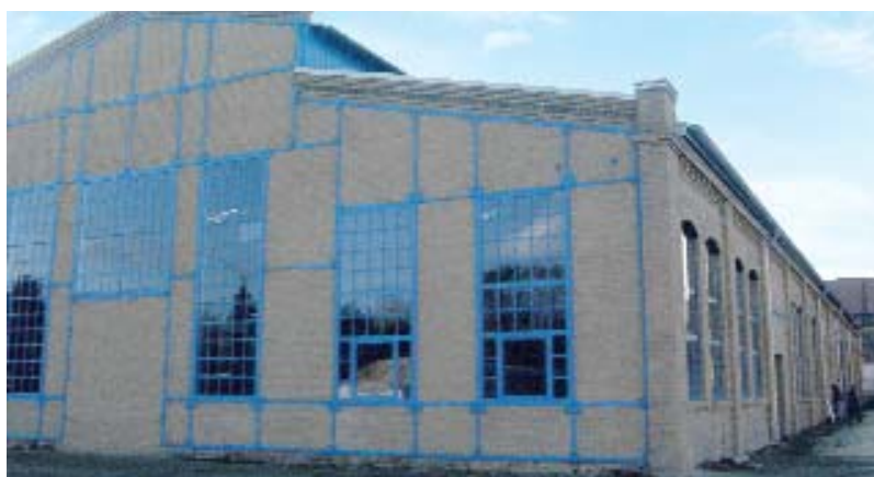
Restored facades for the new foundry model workshop
