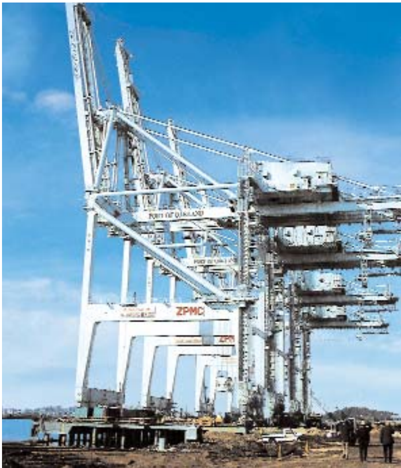
Driven by VEM motors: Port cranes in Oakland (USA)
