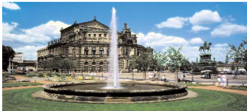
Semper Opera House in Dresden: No disturbances from the stage systems
